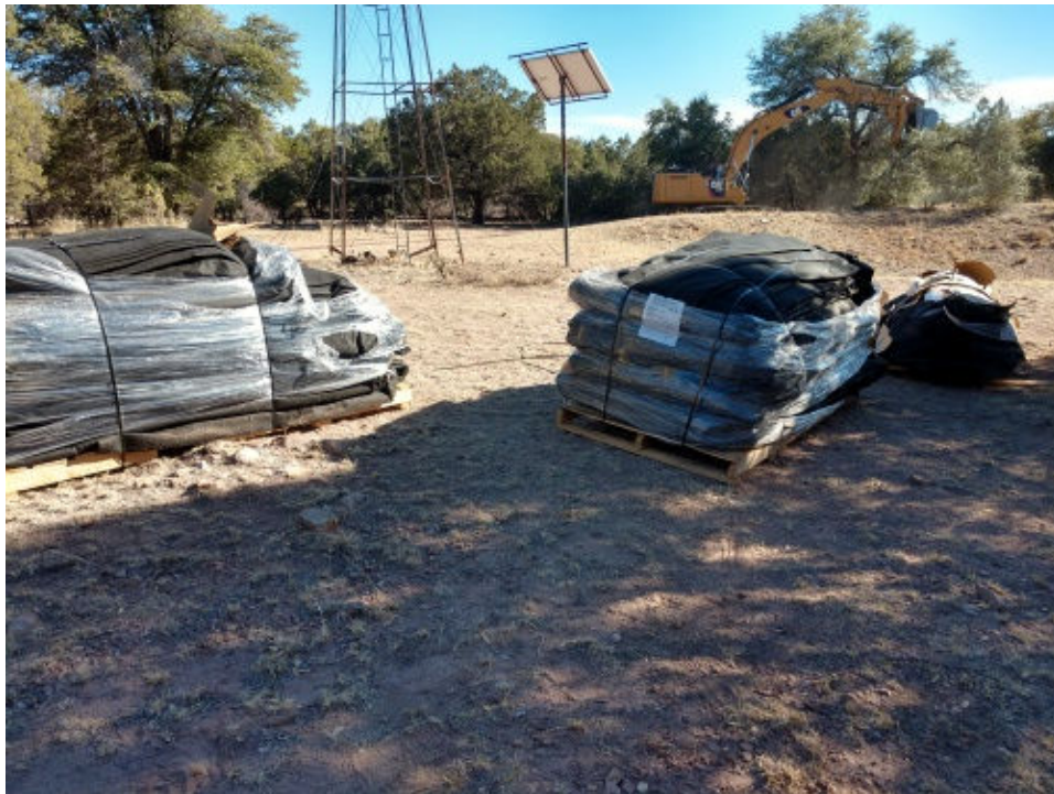
The liner and geotextile are delivered to the project site by pickup truck and trailer so they may be installed.
