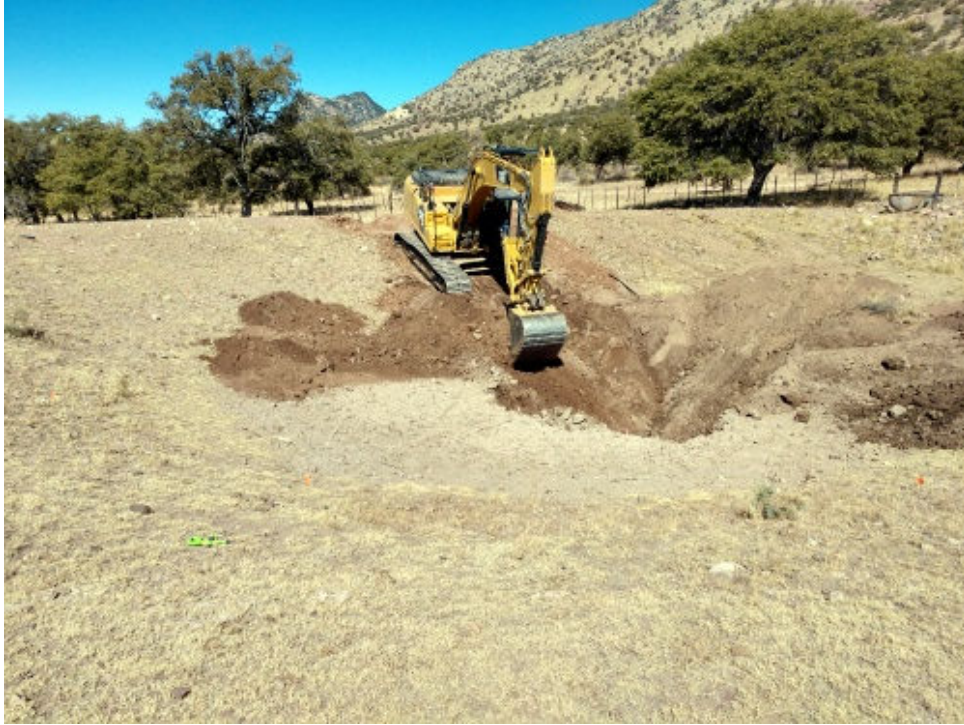
A large excavator is used to dig the basin for the wetland.
