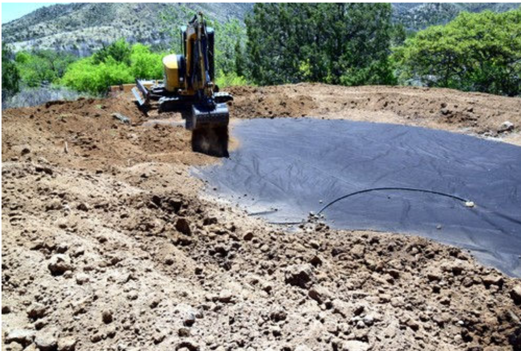
The excavator is used to place soil over the liner and geo-textile pads. Heavy equipment must always be kept off the liner to protect it from damage.
