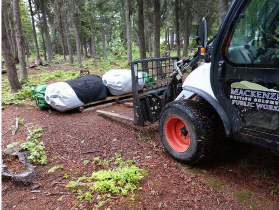
Here a tractor with a forklift attachment is used to move a pallet containing a liner and set of geotextile pads to the wetland construction site.
