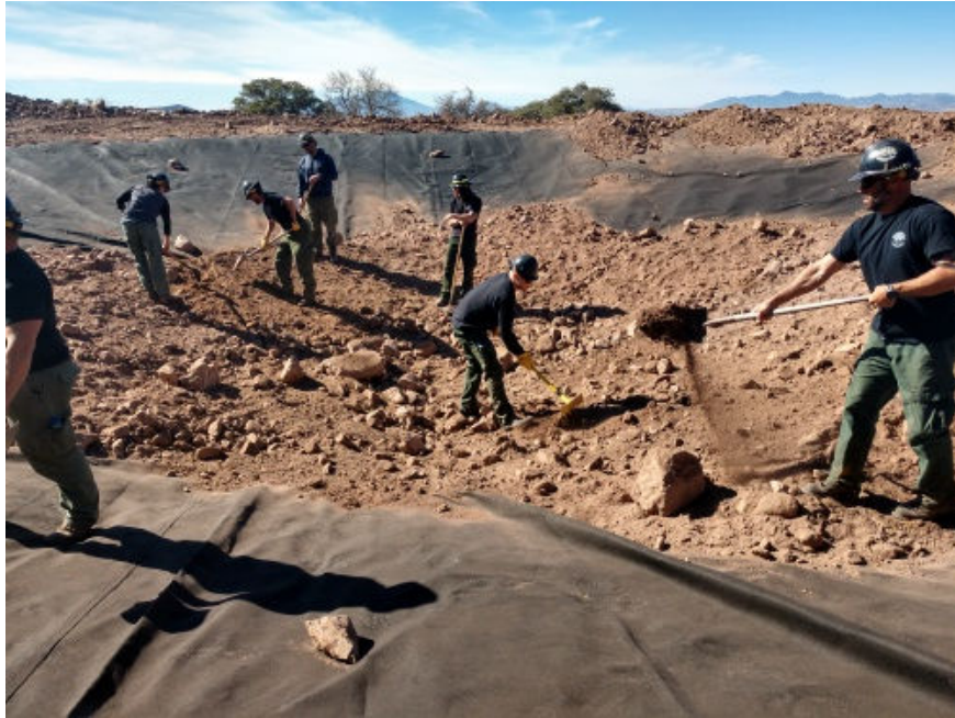
A considerable amount of hand labor is required to cover the liner and geotextile with soil. Heavy equipment must not be allowed to travel over the liner and geotextile.
