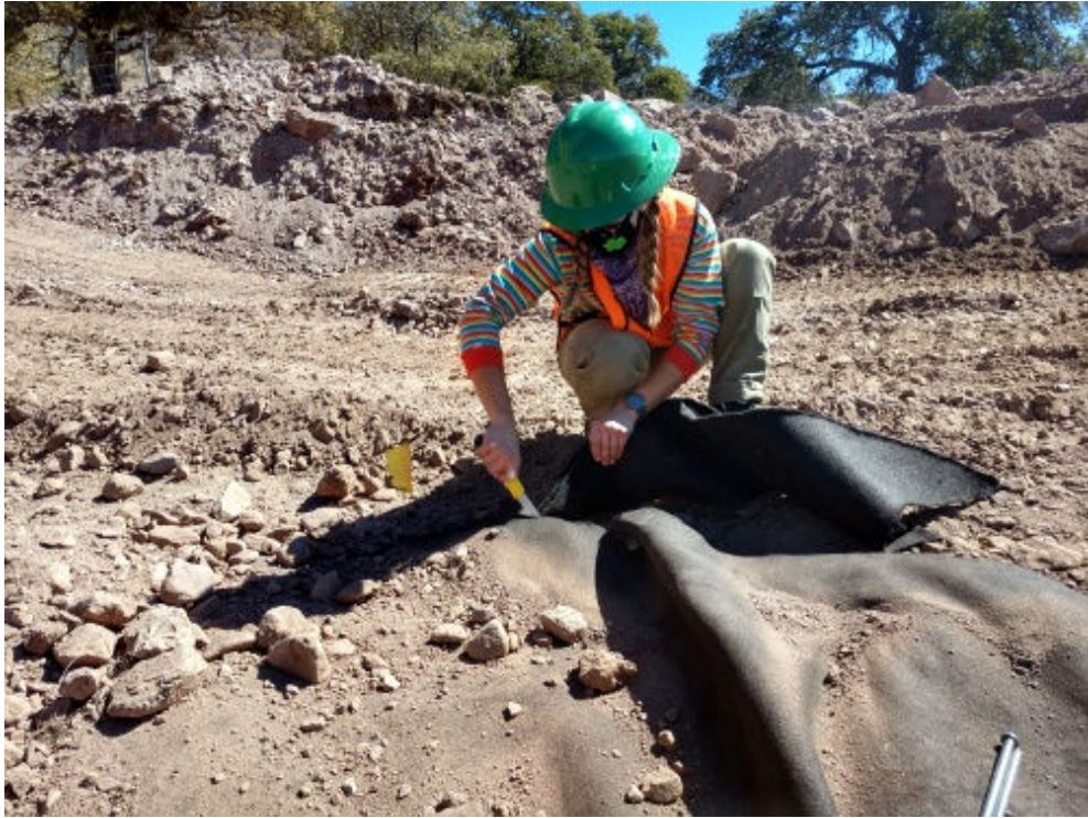
Here excess liner and geotextile are trimmed by hand before covering with soil.
