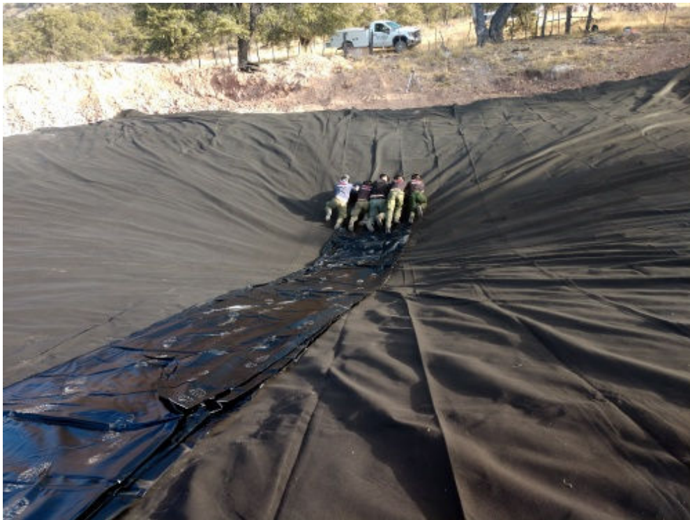
Here a group of Forest Service Wildland Fire Fighters place the liner over a layer of geotextile. The placement of a large liner and geotextile requires the help of at least 15 strong individuals.
