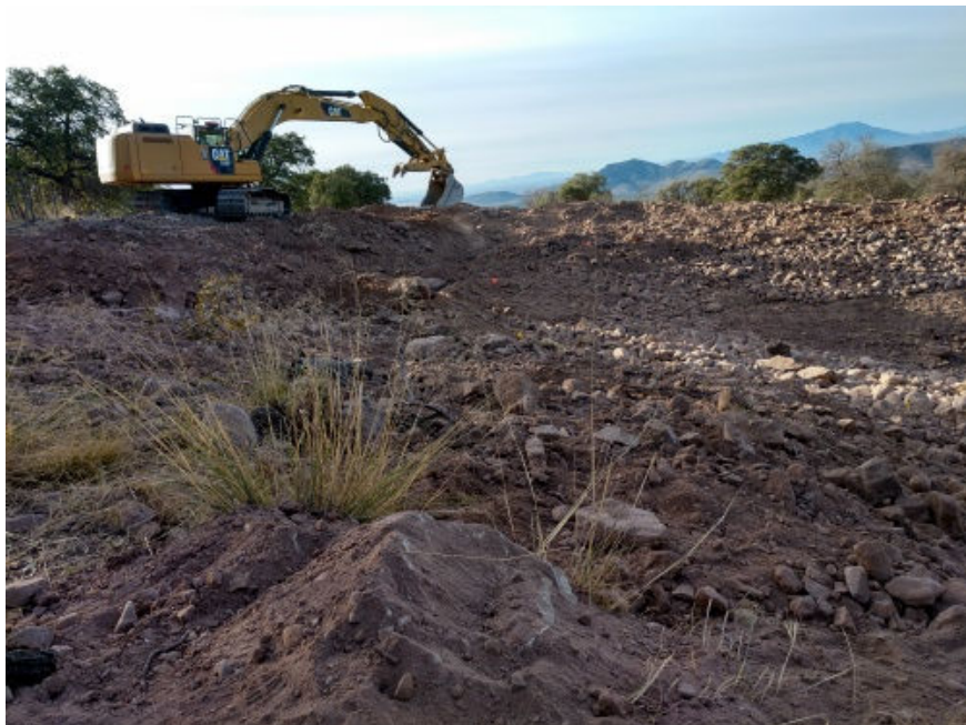
Here the excavator is covering the liner and geotextile with soil. The long reach of a large machine saves time and the need for hand labor.
