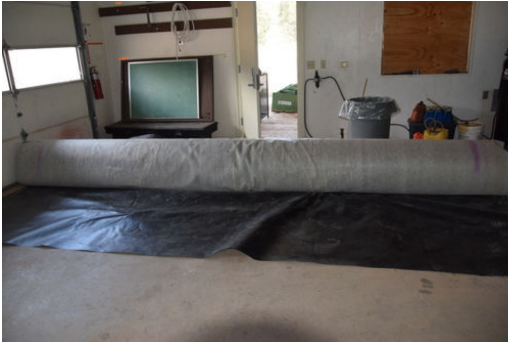
This photo shows a roll of bentonite liner material being stored in a garage. It took 15 people to unroll the material 4-feet. The roll is lifted and moved using a long pipe, chain, and backhoe.
